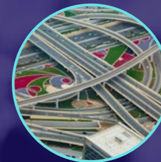
Infrastructure Engineering Zone
